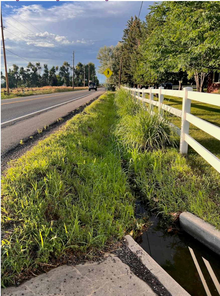
Overgrown drainage channel along Overland.
