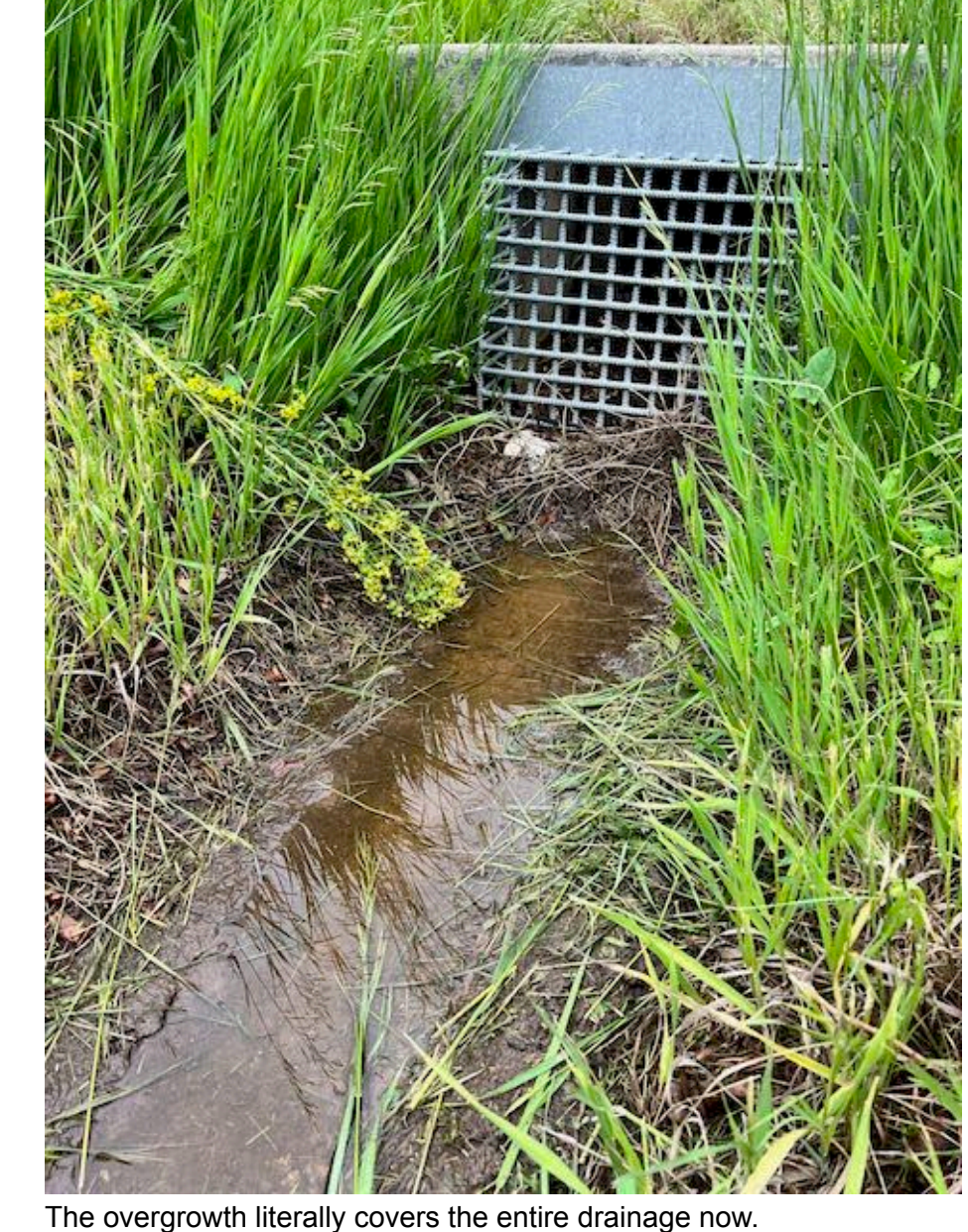
The overgrowth literally covers the entire drainage now.
