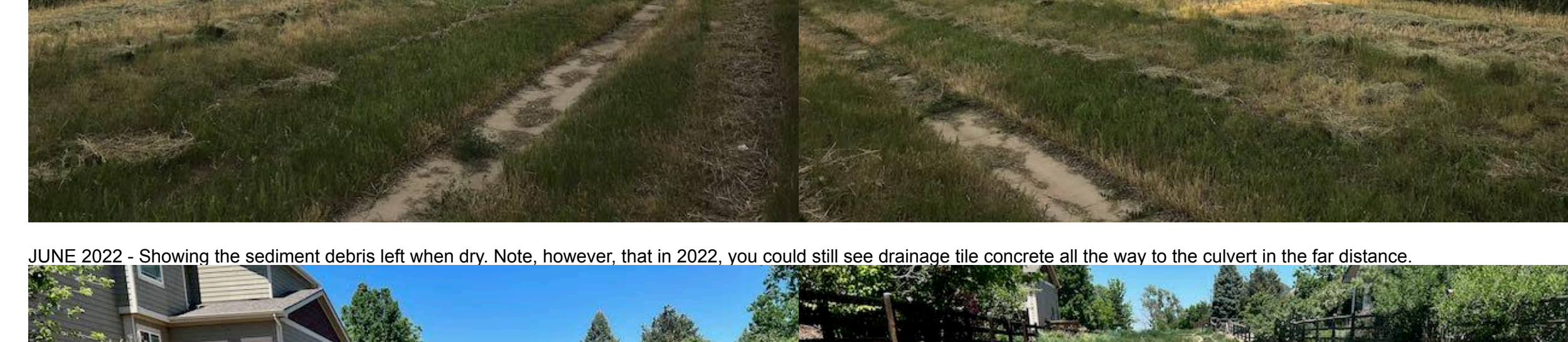
JUNE 2022 - Showing the sediment debris left when dry. Note, however, that in 2022, you could still see drainage tile concrete all the way to the culvert in the far distance.
