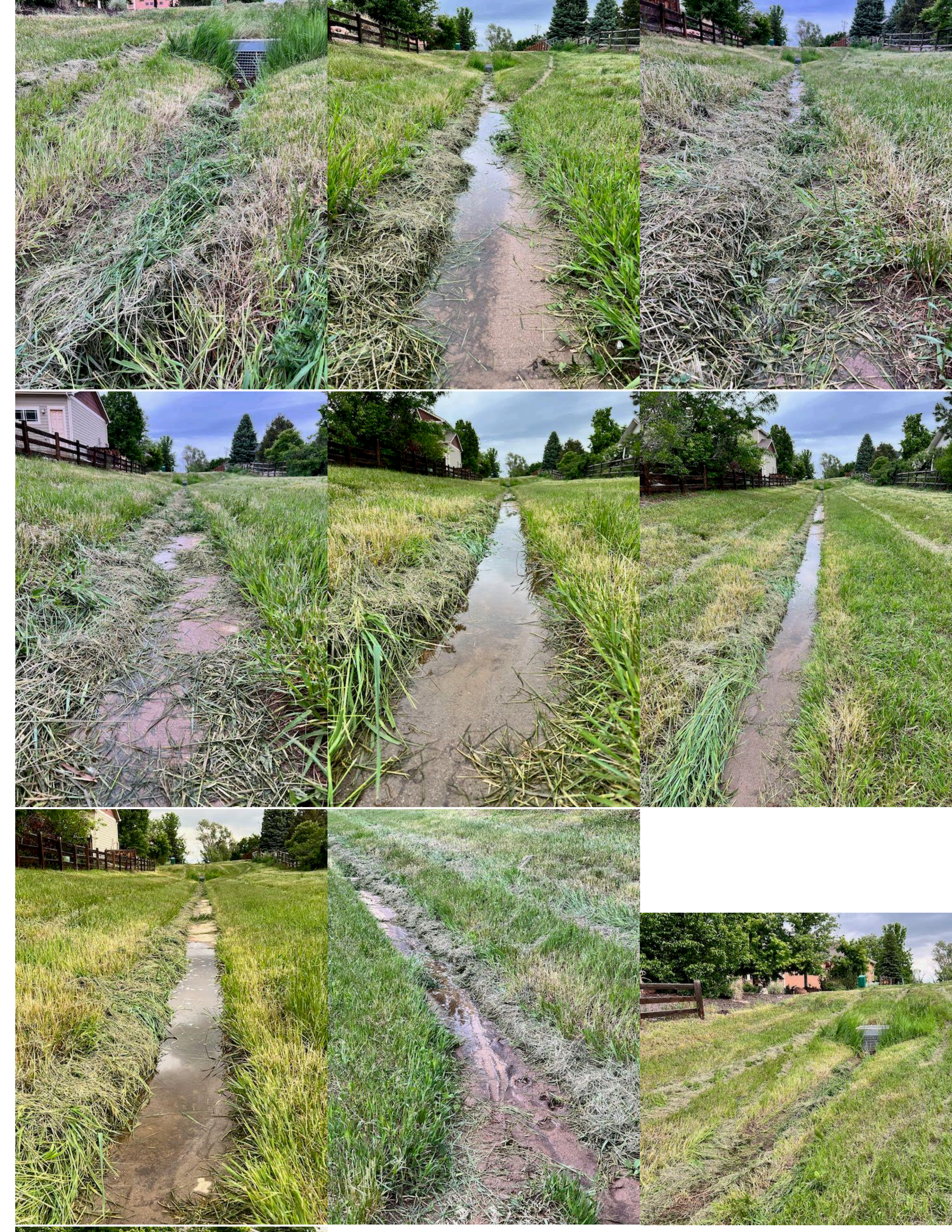
The overgrowth literally covers the entire drainage now.
